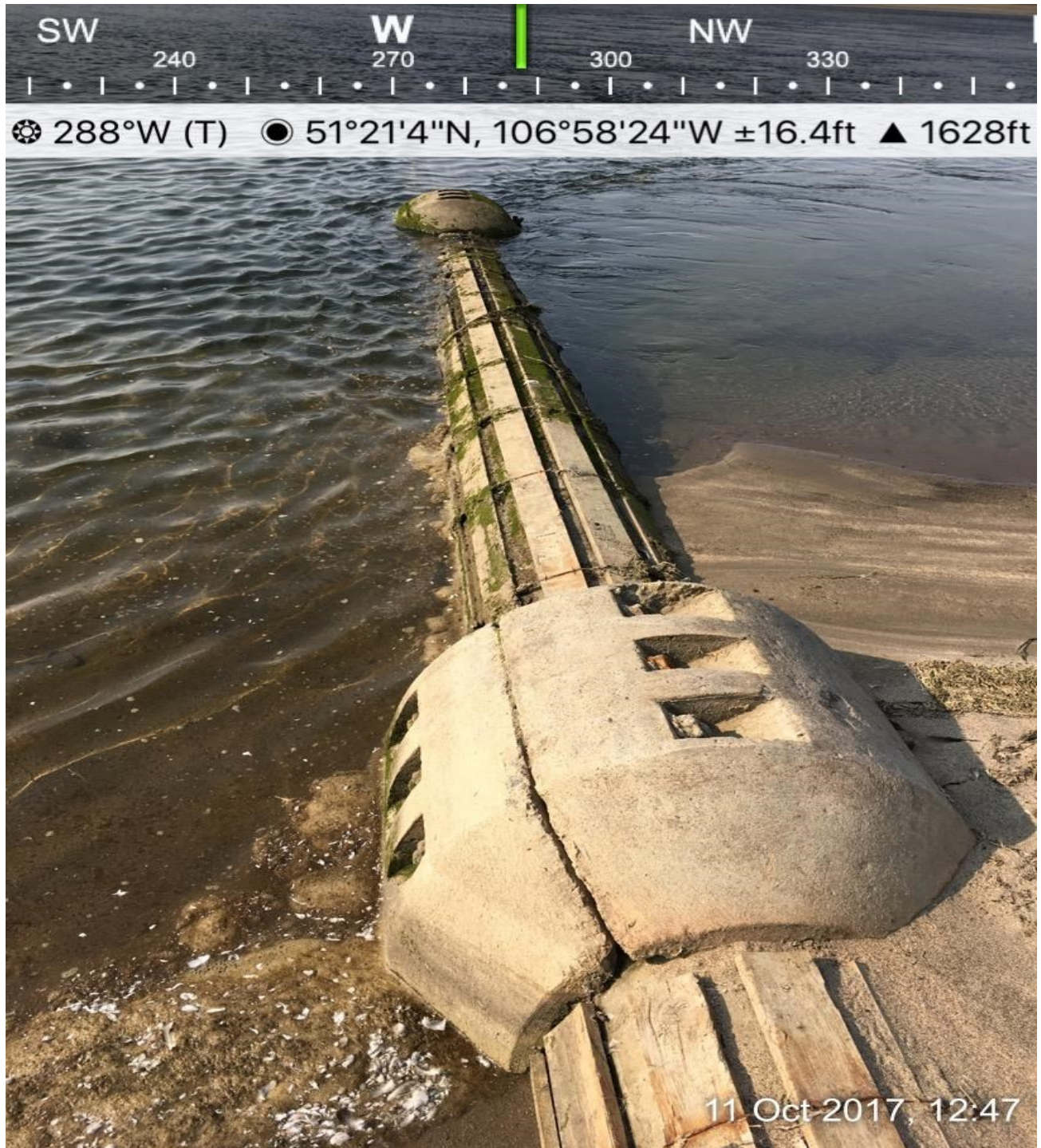
East end of South Saskatchewan River existing pipeline.
