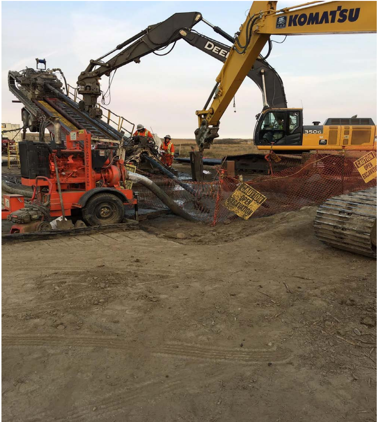
Directional Drilling at South Saskatchewan River
