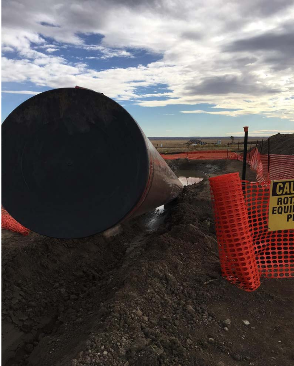
Pipe that was pulled thru (RD 34)
